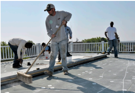
Workers install a white roof on a museum building at University of Central Arkansas. Photo: UCentralArkansas
